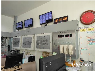
Graphic Annunciator Fire Alarm
