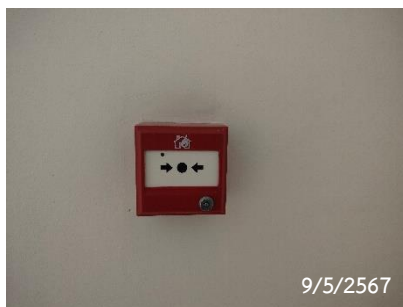
Fire Alarm Manual Station
